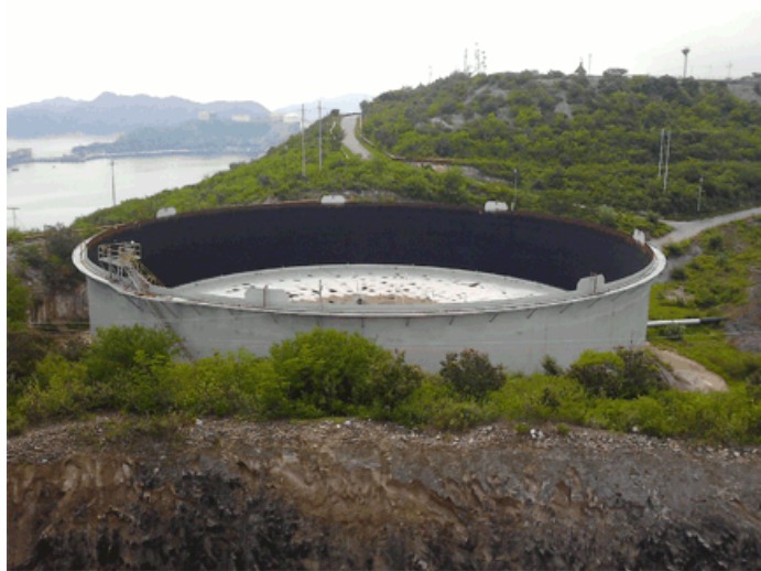
Figura 4.2 Tanque 260x2, Terminal Marino Guaraguao
