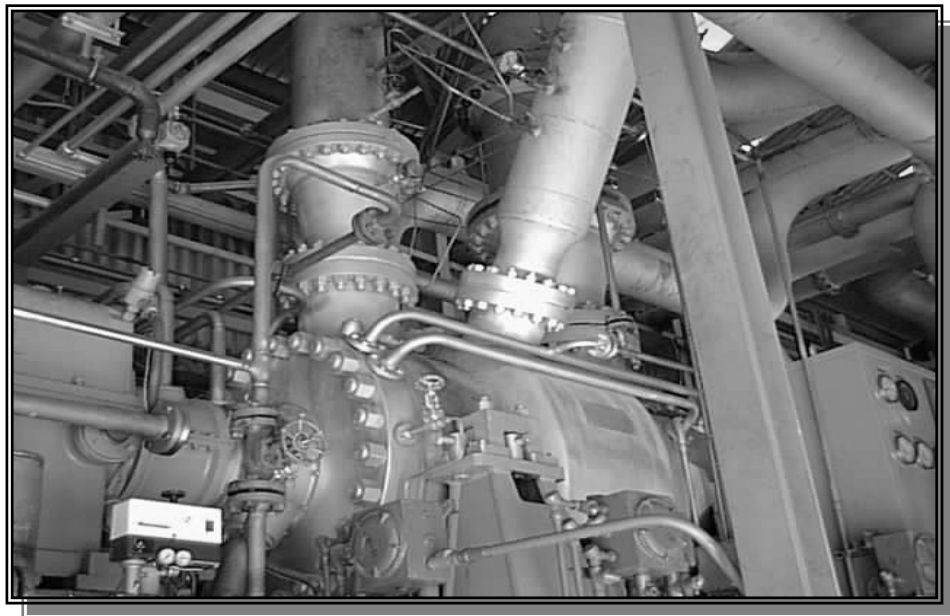
Fig. N° 2.5 Compresor de gas residual [3]
