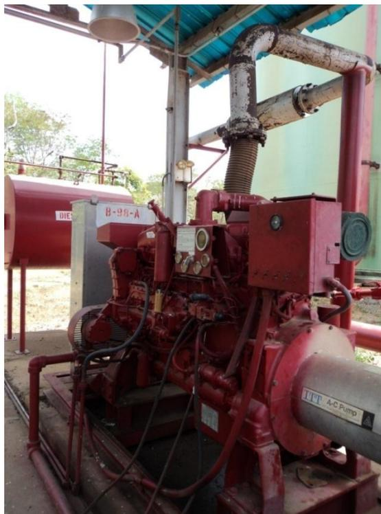
**Figura 4.6. Bomba Principal Diesel (B-98 A)**
