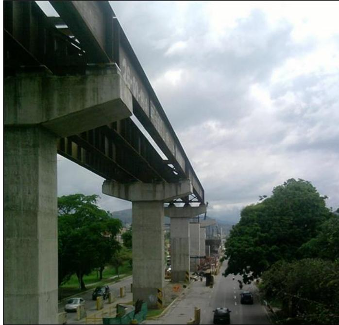
Figura 53. Estructura mixta, Metro Guarenas-Guatire
