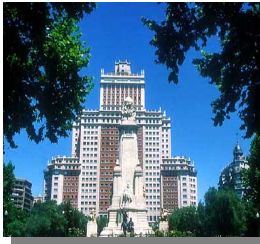
Figura 1. Vista del Hotel Crowne Plaza Madrid City Centre.
