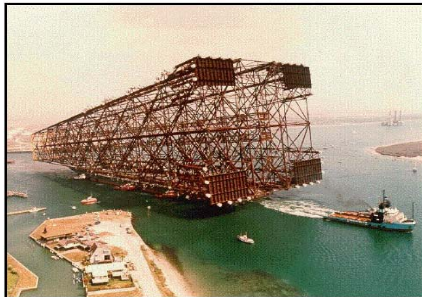
Figura 2.2 Transporte de Jacket. Fuente: Shell Deepwater Development Systems Inc.2005.
